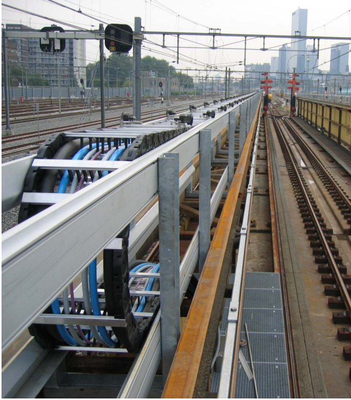
example train wash: free weathering extreme influence of media (detergents) travel 180 m
